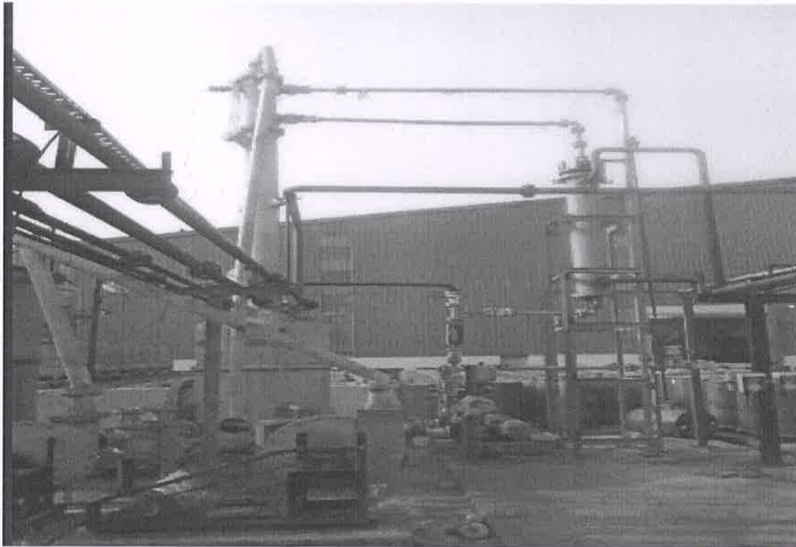
10. Two stage scrubber installation for process vent in liquid Plant.
